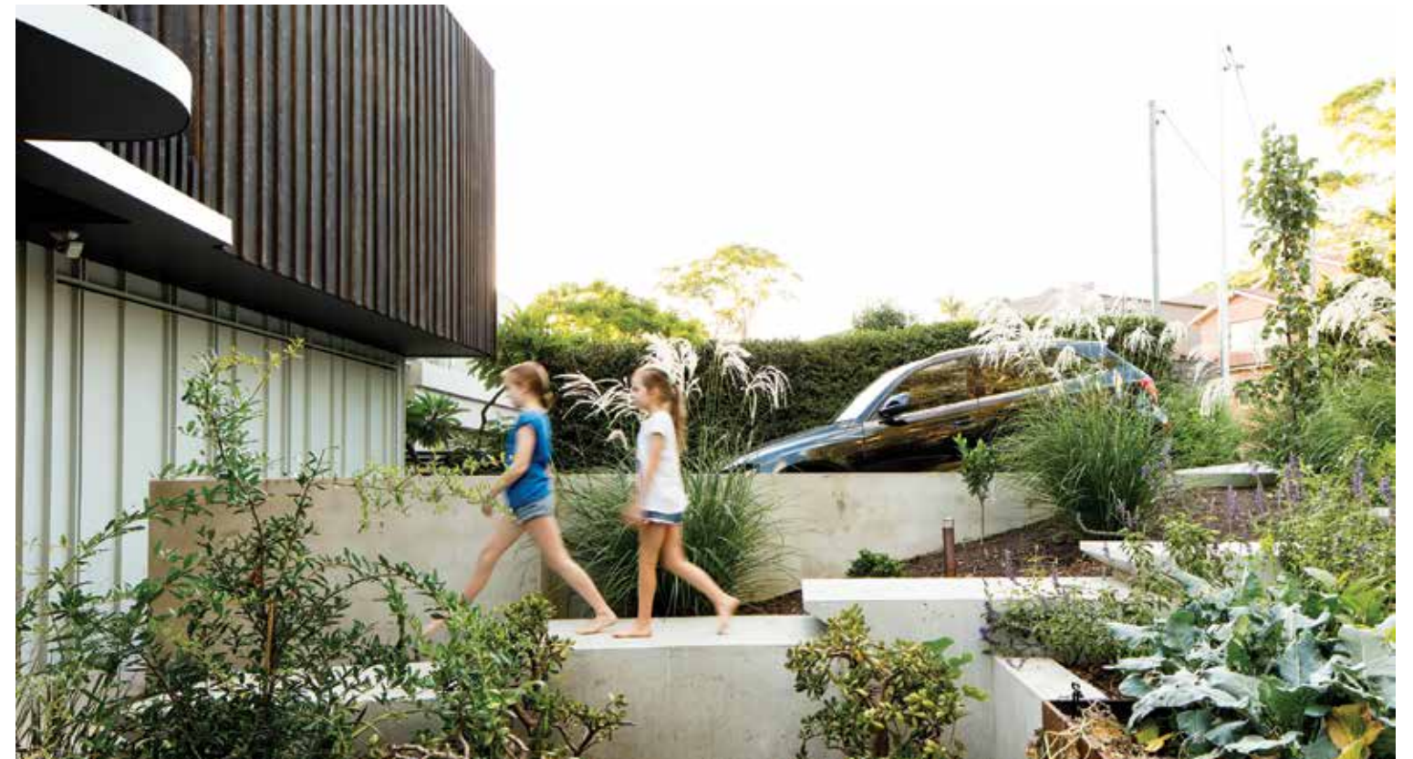
The house is entered via a pathway that steps down through the front garden.
